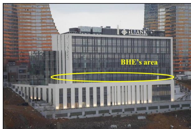
Fig.1. General view of Atasehir Building
