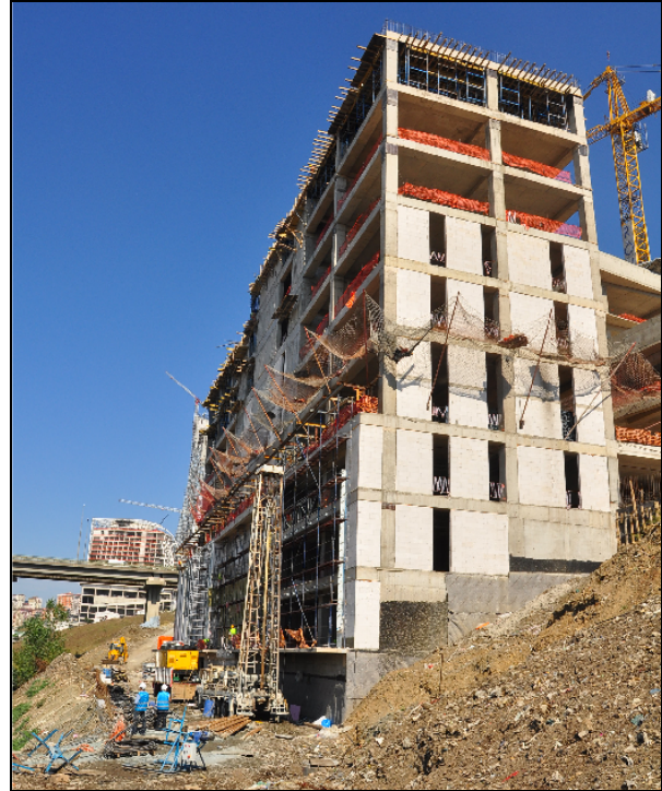
Fig.4. General view of drilling stage
