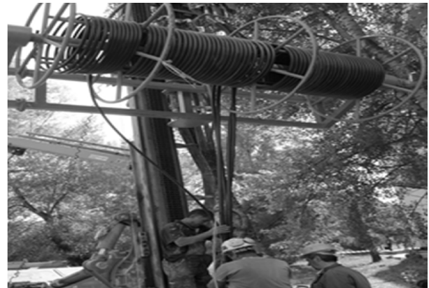
Fig.8. Inserting the HDPE tubes in the perforations
