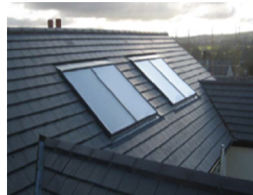
Fig.4. Roof integrated flat plate BISTS for Solar Water Heating
