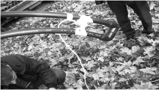
Fig.5. Mounted temperature sensor in the lower part of the U-tube
