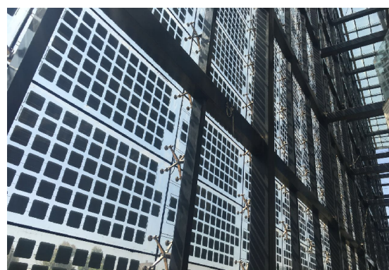
Fig.5. The inside view of the PV curtain wall
